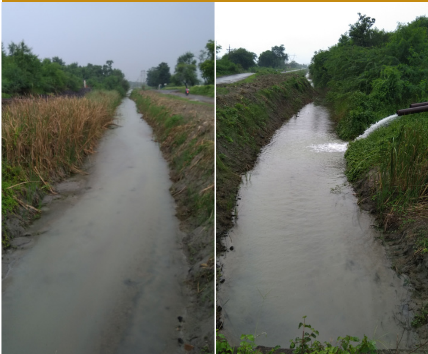
FIGURE 15: PHOTO SHOWING FLY ASH LADEN WATER BEING DISCHARGED INTO A CHANNEL FROM THE KHAPARKHEDA ASH POND. THIS CHANNEL IS UNLINED AND WATER WILL SEEP INTO GROUND WATER FROM THIS CHANNEL AND ALSO POSSIBLY CONTAMINATE OTHER SURFACE WATER BODIES | PHOTO: SHRIPAD DHARMADHIKARY/MANTHAN ADHYAYAN KENDRA | YEAR 2021
