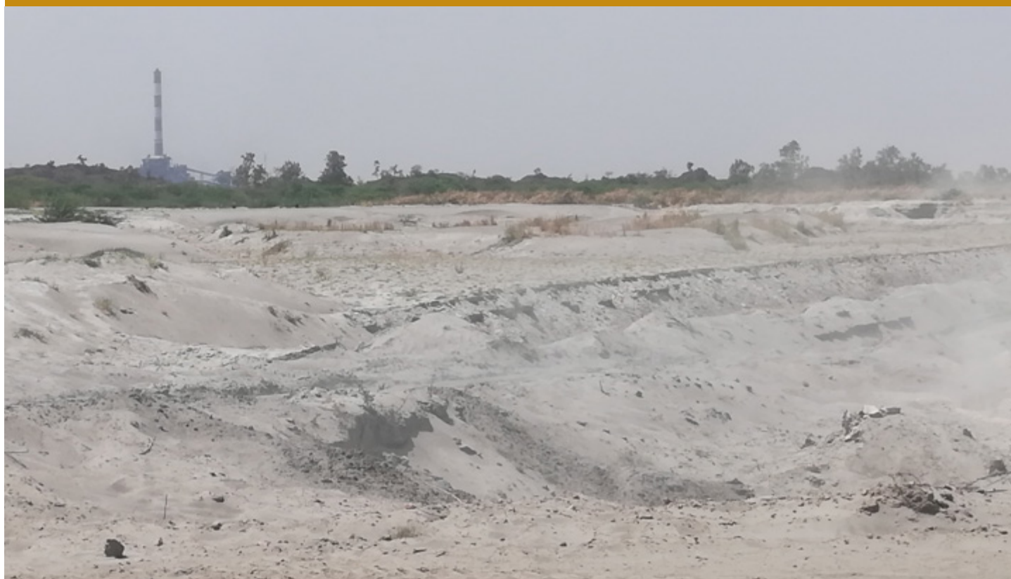
FIGURE 14: DRIED SECTION OF KHAPARKHEDA ASH POND AND ASH BEING BLOWN BY THE WIND. YEAR 2019 | PHOTO: SEHR RAHEJA/MANTHAN ADHYAYAN KENDRA
